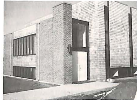
Front Entrance to the Twin Pines Baptist Church building.
