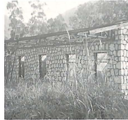
Rural Health Center Under Construction
