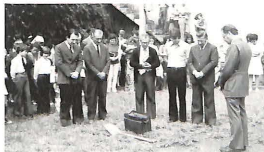
The groundbreaking service for the new building at Caxias do Sul took place on Dec. 30, 1973.
