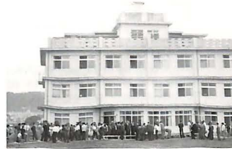
The Dormitory-Dining Hall building at the time of the dedication in 1968.
