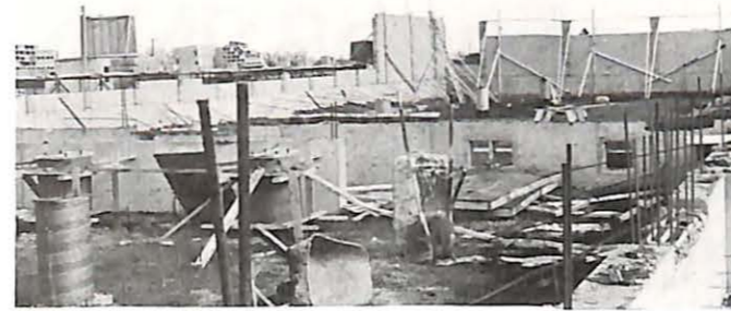
The North American Baptist College under construction.
