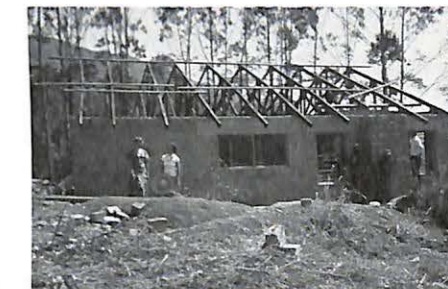
A new missionary residence at Mbu under construction.
