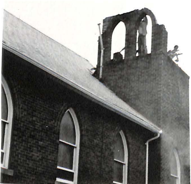
Remodelling of the deteriorating steeple.
