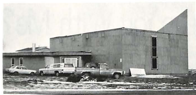
The church edifice under construction.
