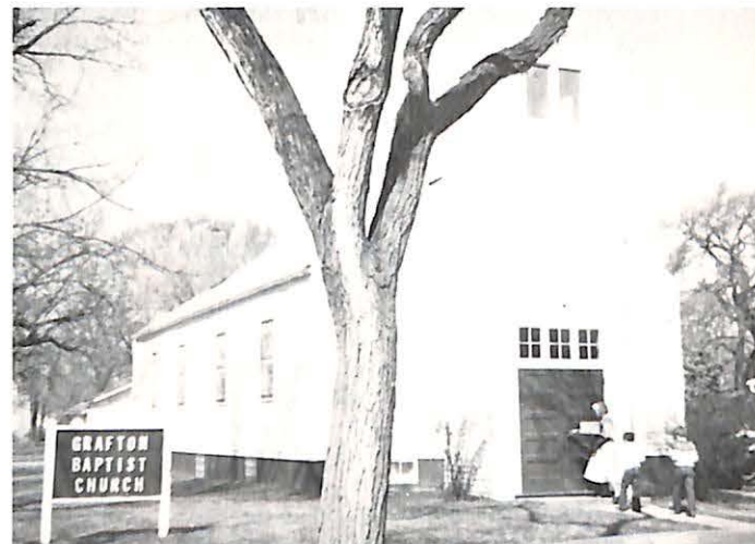
Present place of Grafton Baptist Church while the congregation looks for more adequate facilities.
