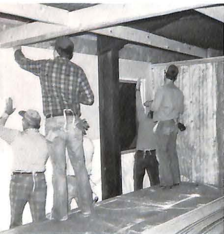
Members of Metropolitan Baptist put up plaster board
