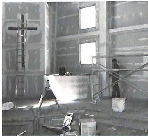
The sanctuary under construction
