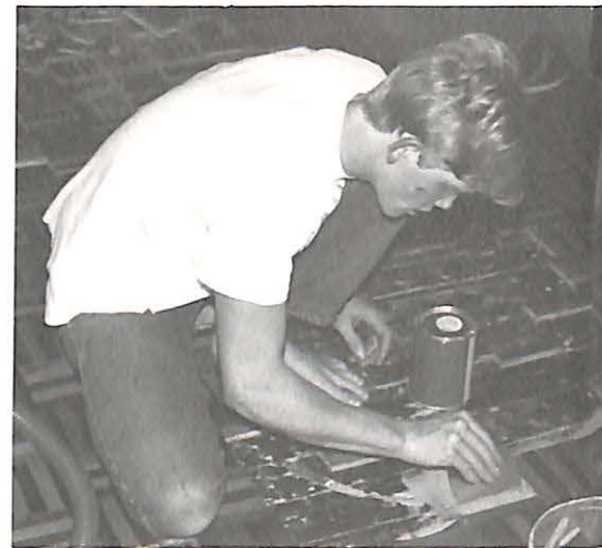
Repairing parquet floor in the study of the mission home in Caxias do Sul.
