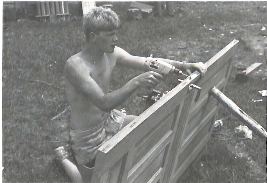
Phil mounts hardware for door for cook's new sleeping quarters at the State Baptist Camp in Santa Maria.
