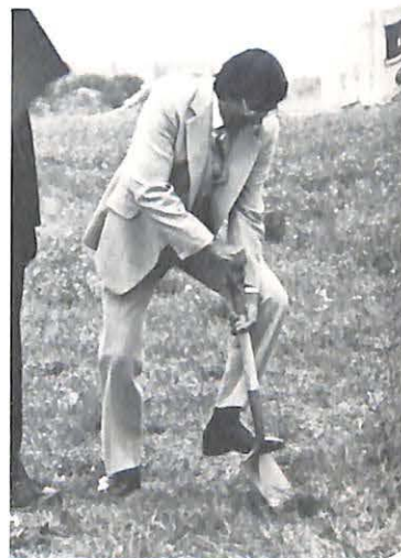
One of the original core members of the congregation, John Machado, breaks ground for the new church.
