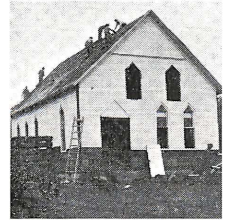
Dismantling the old church building to make room for the new one. For 45 years this building was used and became a place where many found their Lord. Christians were edified, Christian fellowship was practised, and the Church unitedly made earnest prayer.
