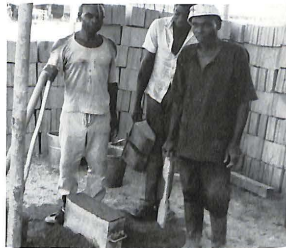
The construction workers make bricks for the Home Economics Centre, Mutengene, Cameroon. Money is provided through Baptist World Aid as well as the Women's Missionary Fellowship for this construction.
