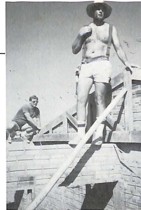
Construction leader Terry Jorgensen (standing) and electrician Cal Erickson begin placing the rafters on the parsonage.
