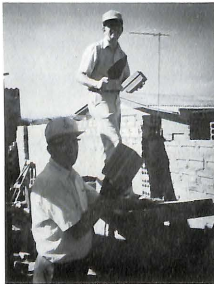
Leroy Caswell and Dale Cundall make progress on the parsonage wall.
