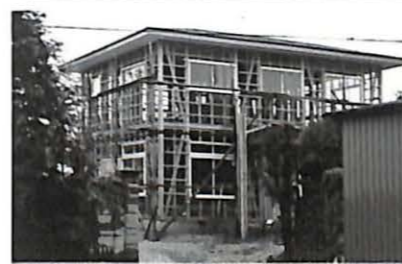
A missionary home as it was under construction in Nagoya, Japan.
