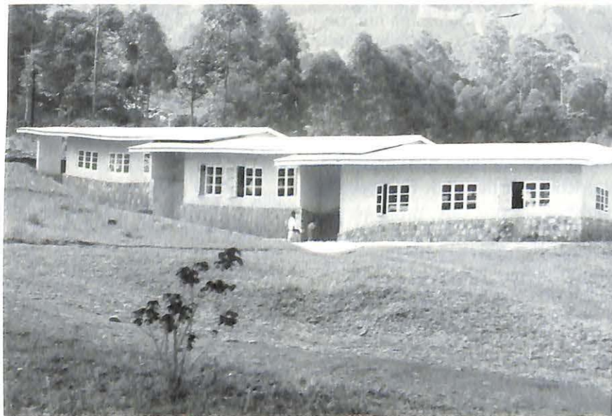
The main dormitory at Baptist Comprehensive College, Njinikijem-Kom, Cameroon, was built with contributions to the Capital Funds Campaign.
