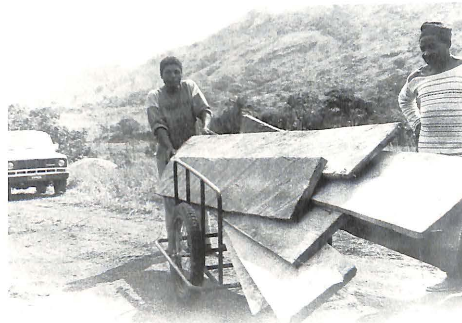
When the motorable road ends, building materials are transported on two-wheel carts.
