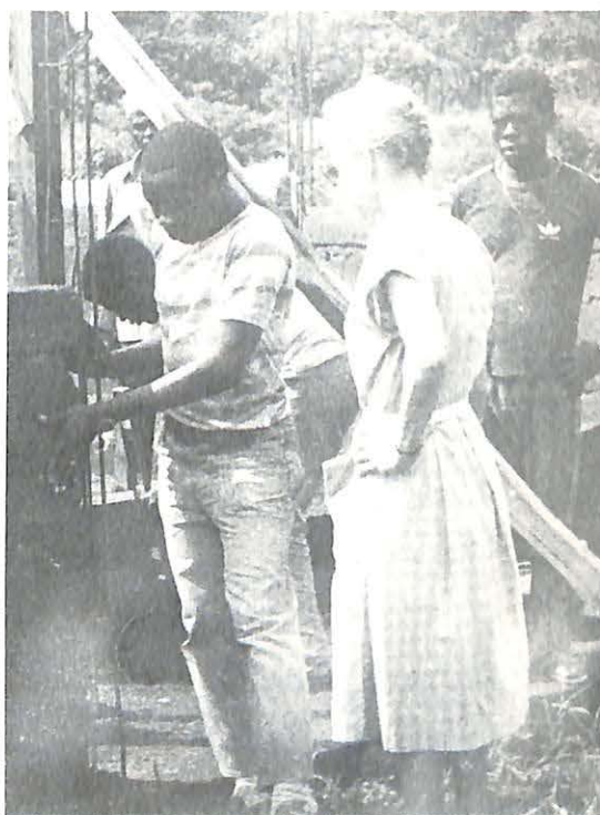
Workman prepares metal support for walls of mud brick homes.
