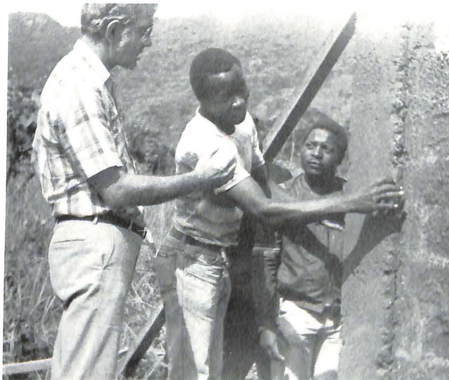
At the Bwabwa building site, Dr. Oryn Meinerts (left) encourages Pastor Emmanuel Nsah, assistant building coordinator.
