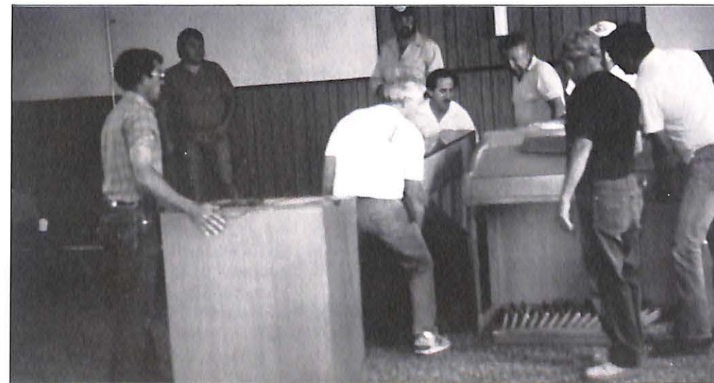
They stripped the sanctuary to begin remodeling. The ceiling was lowered, and a new one of aspen put in place; walls were torn down, redone, painted and/or paneled; a new hot water heating system replaced the old noisy blower; new carpet provided a unifying element and a baptistry was installed — the first in the Church's history. The Church now has an open cheerful look.
