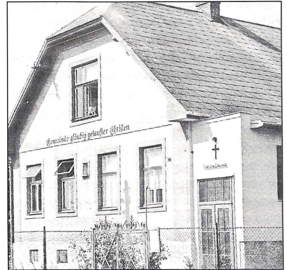
The Baptist Chapel at Essling, Austria, meeting in a former residence.
