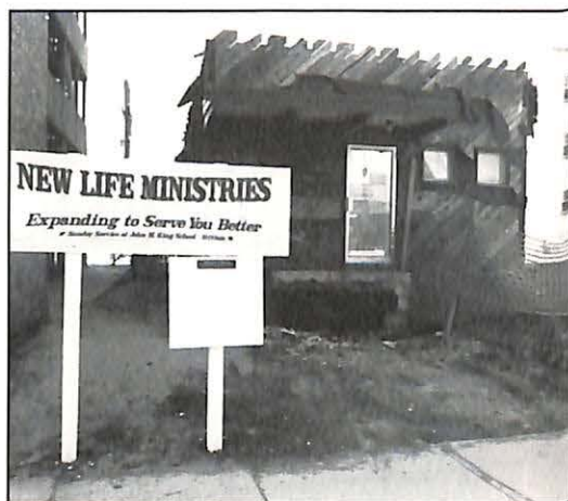
Pastor Lehotsky was the first to pick up a hammer and begin knocking down the walls of the 20- by 40-foot building New Life had used in its metamorphosis of ministry.
