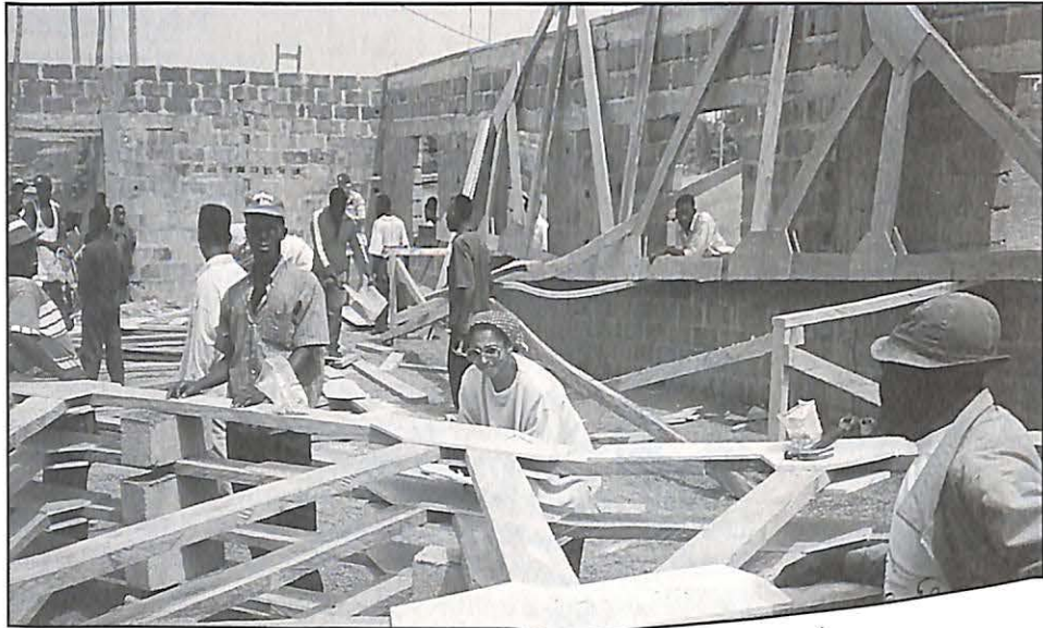
Many hands make light work as Africans and Canadians unite to build a roof.
