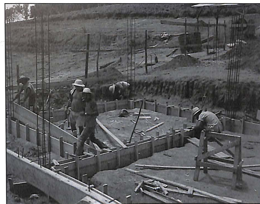
A foundation was laid prior to the coming of a volunteer team from Canada to construct the first CHAIN of Love home.
